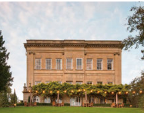
South West Bailbrook House Hotel, Bath
